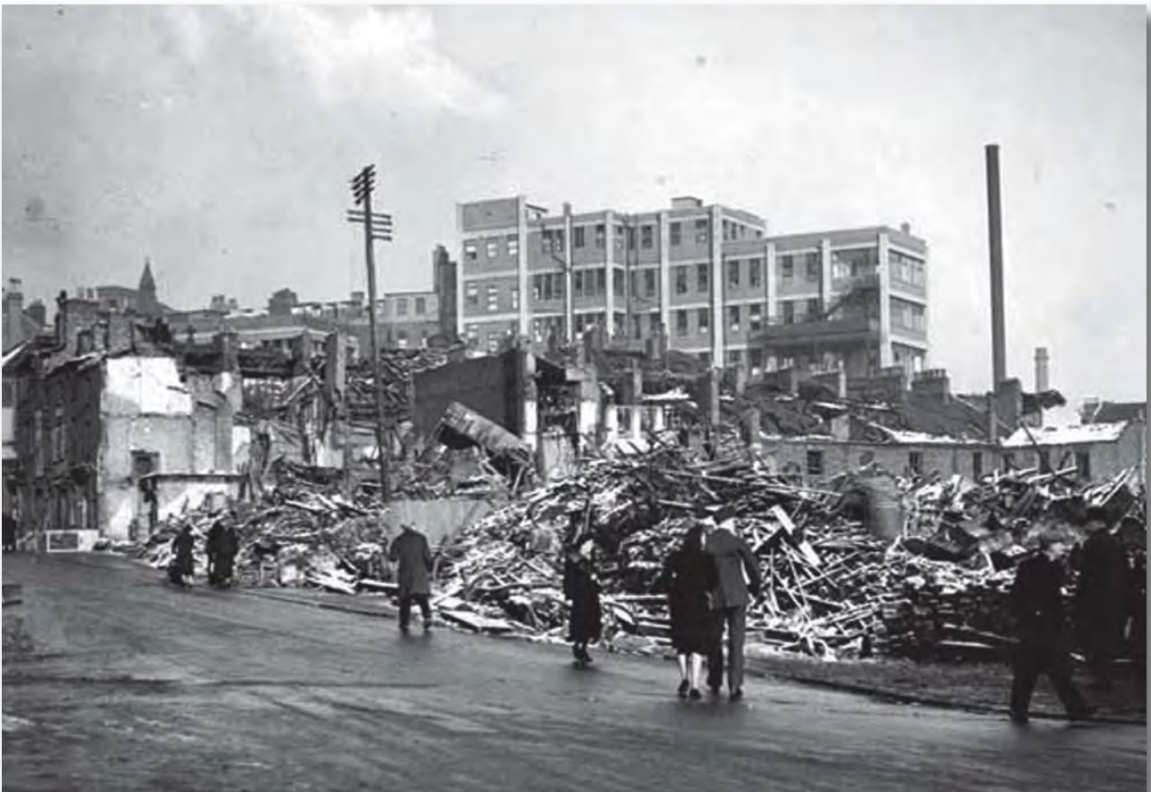
Fitzwilliam Street, showing air raid damage with Royal Hospital in the background.
